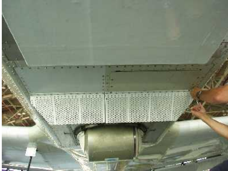
Figure 3: Detail of center area of bomb bay and baffle. Note the hinged door on the port side (right side of the picture). This door appears to open out normally, but here is pinned down by the baffle hardware. If the door were open and the baffle were removed, the resulting aperture would be 24" wide \times 25" in the direction of flight.
