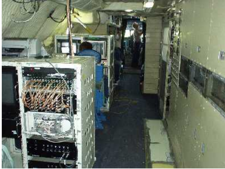
Figure 8: A view of the instrument racks from the middle of the large cabin area, looking forward. Two instruments are visible, both on the left (port) side: ESTAR (closest to the observer) and PSR (just behind ESTAR).
