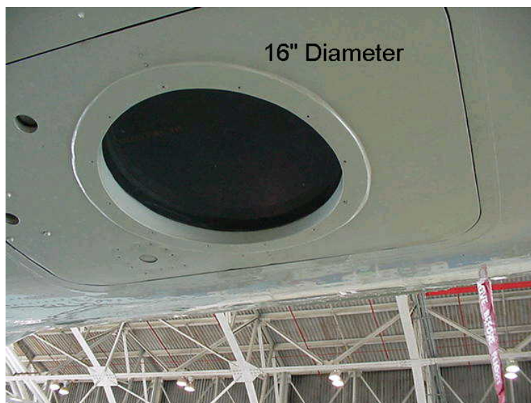
Figure 11: Middle Nadir Optical Port, located a few feet to the rear of the forward port (Figure 10). Picture courtesy of D. Easmunt, WFF.
